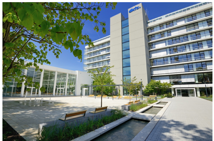
DKFZ main building: The German Cancer Research Center (DKFZ) in Heidelberg is one of 15 oncology centres of excellence in Germany. © Tobias Schwerdt
