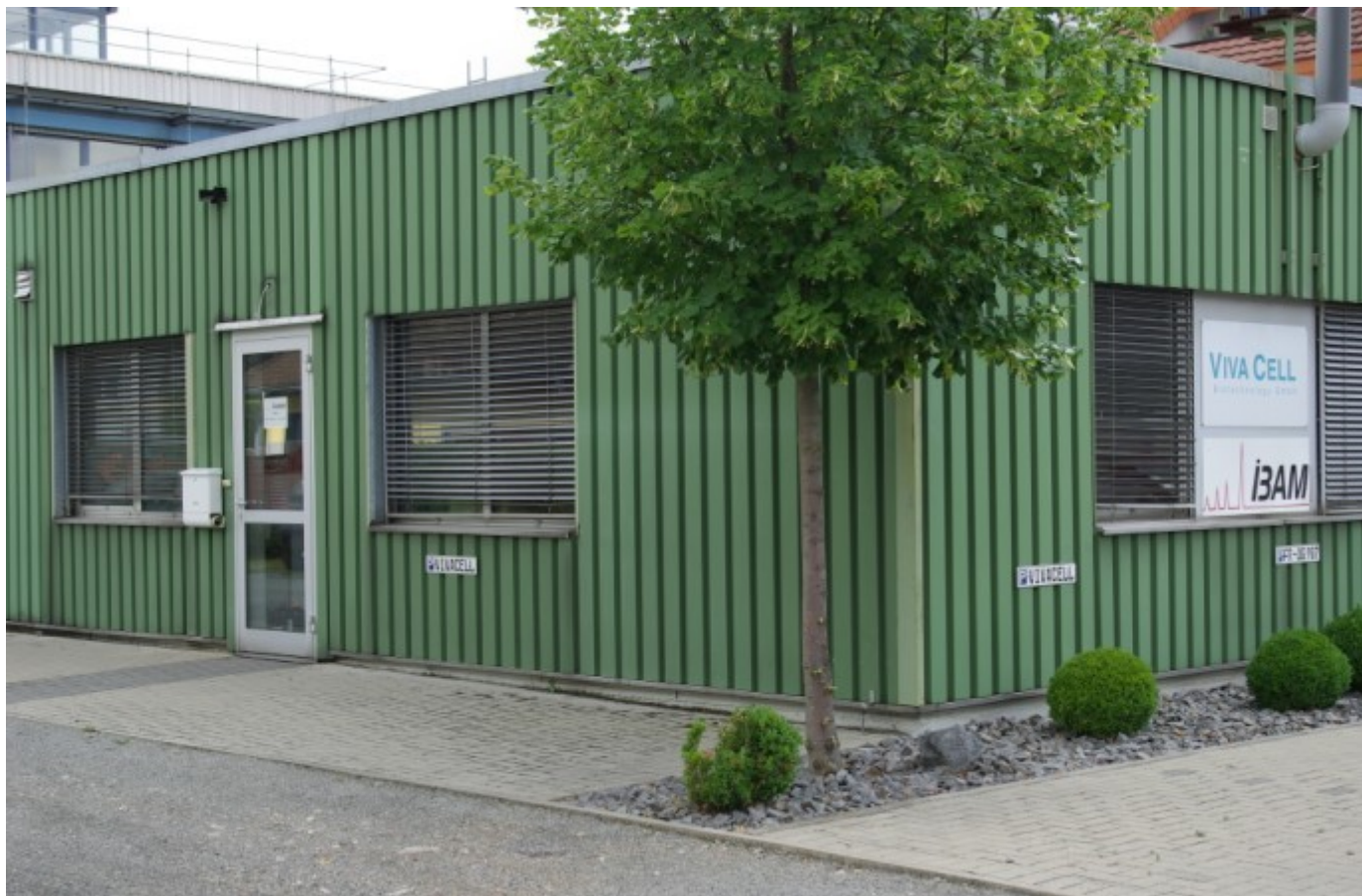
The IBAM GbR headquarters are located in the same building as Vivacell Deutschland © IBAM GbR
